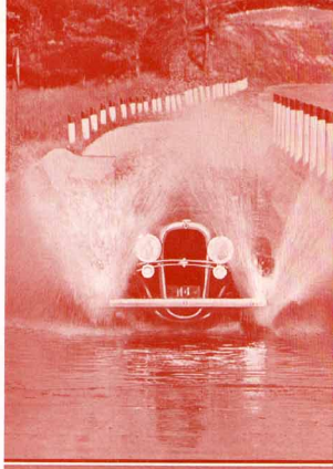
Every possible test which an automobile may encounter in actual use is given Oldsmobile on the General Motors Proving Ground. Here is the "bath-tub."
