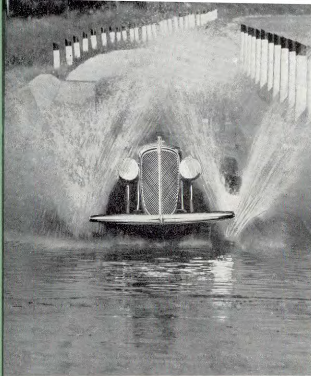
The "Bathtub" . . . an automobile has to be absolutely weather-proof to pass this rigorous test.
