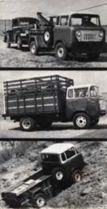
Custom-built wrecker combines with "Jeep" FC-170 and push bumper to produce this indispensable unit for garages and service stations. The plus-traction of 4-wheel drive means more pulling and pushing power on or off the road. Turn radius 21 ft., 10 in.
