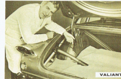
Valiant's gasoline intake line extends well into the trunk compartment, taking up valuable luggage space. Rambler's intake line does not enter the trunk compartment.
