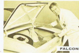
Sound-deadening material that is merely thrust into the sides of the Falcon trunk compartment is short-cut construction. Rambler sound-deadening materials are built-in.
