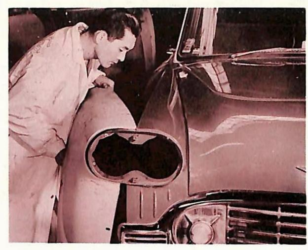
Practical two-piece construction allows for removal of entire fender assembly or just outer half from inner portion without disturbing other parts.
