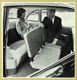
The twin, forward facing auxiliary seats form one complete seat and provide adequate room for three adults with limousine comfort. Extra-wide (132.08 cm.—52 inch), the auxiliary seats are fully cushioned with sturdy, shoulder-high backs. When not in use, they fold flat against the back of the front seat and their base support forms a footrest for back seat passengers. Upholstered in a wide choice of long-wearing luxurious fabrics.
