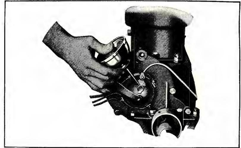
Oiling the Ford Commutator. (Cut No. 19)
