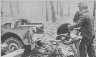
The Universal "Jeep" with special power take-off in the rear, is a mobile power unit, always ready for any farm chore from
