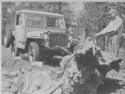
A capstan winch is optional equipment available for the "Jeep". It is mounted between the bumper and radiator and driven through a propeller shaft. Designed for 5,000-pounds pull, the winch helps pull stumps, drag out mired equipment and other vehicles.
