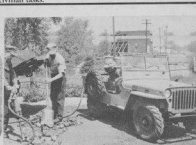
The "Jeep" wants to work with crews of street and sewer departments, public utilities and transportation companies. Here the "Jeep" with power take-off furnishes power for a compressor for pneumatic tools.
