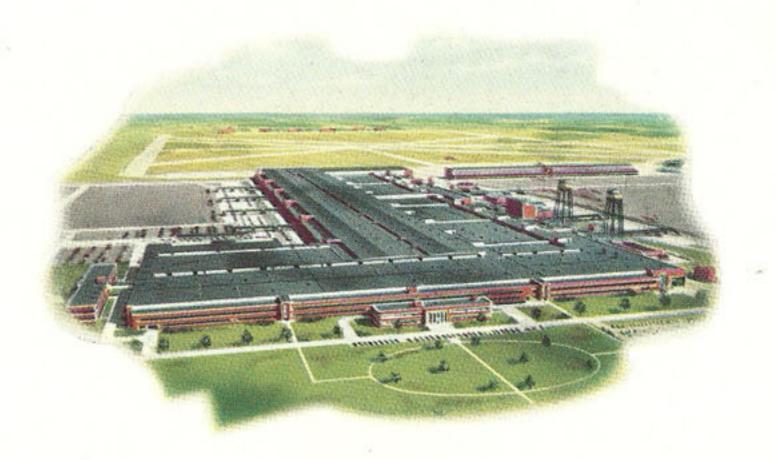
Willow Run was built during the war for the mass production of B-24 bombers. One of the largest industrial plants in the world, it has more than 80 acres under a single roof. Its main building is over 3,000 feet long! Here the automotive technique of line production was applied to giant aircraft—finally reaching a peak of sixteen \$250,000 war planes a day—one every working hour! Willow Run contributed mightily to the victory of American arms in every theater of war. But after V-J Day,
