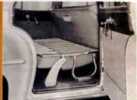
Note the uneven, wavy floor in the Carry-All here at the front. The back section slopes to the rear of the car. Observe how the front floor section rests on the padded arm rests of the folded rear seat, and finally notice that the cargo carried comes in direct contact with the vinyl upholstery on the back of the front seat.
