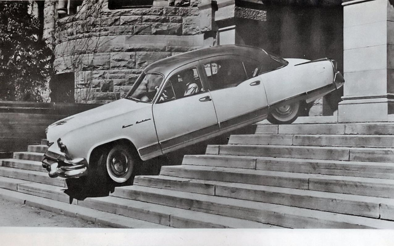
A 1953 Kaiser Manhattan glides down a flight of stone steps in a dramatic demonstration of the effectiveness of Kaiser-Frazer's new "full control" power steering. With conventional unassisted steering, the shock of the eight-inch steps would twist the wheel from the driver's hands. Simplest and least expensive yet introduced, the Kaiser hydraulic unit absorbs road shock and provides virtually effortless steering control at all speeds.
