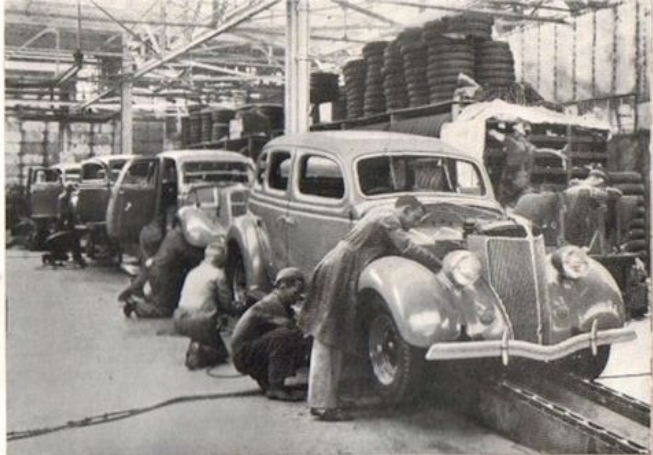
(Above) Converging on this focal point—Body and chassis finally complete the last stage of their journey. The multitudinous operations carried out in every portion of this vast modern factory culminate on the final assembly line. From this line vehicles are driven off under their own power ready for delivery.
