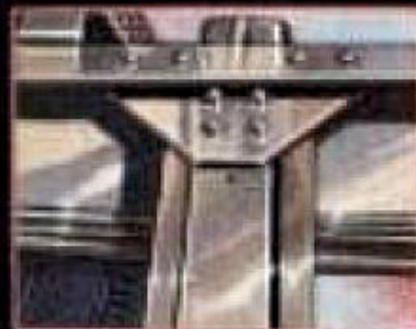
Heavy frame with coil roll 10" x 2" x .312" plus .187" reinforcement
