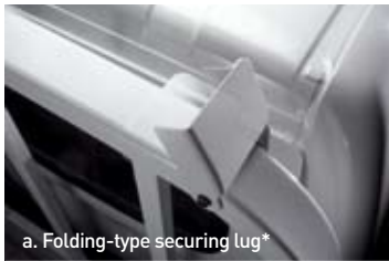
a. Folding-type securing lug*
