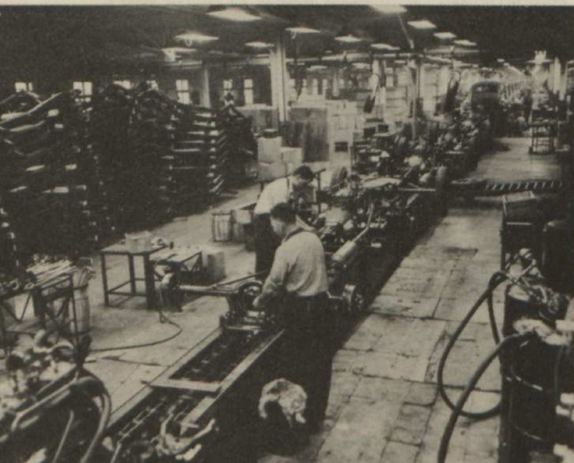
The start of the Nash final assembly line. Bodies enter the line in the foreground.
