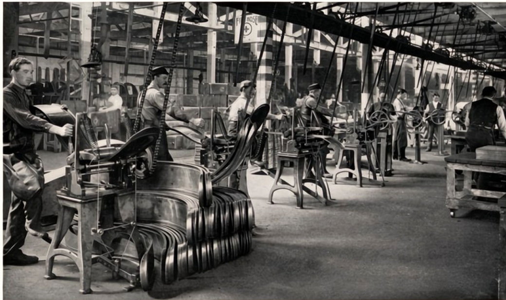
The Jeffery fender department. All sheet metal parts of Jeffery cars are made in a department so large in equipment and capacity as to constitute a factory in itself
