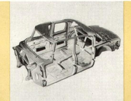
The same box-section design used in the Marshal's frame construction is the secret of its safety-built body. Liberal use of this pound for pound strongest structural design, together with heavy-gauge metal throughout, gives ample assurance of standup stamina and extra safety, no matter how rough the going or fast the action. Cushioning this cradle of steel and the box-section frame are some 300 tiny body and chassis vibration dampeners.
