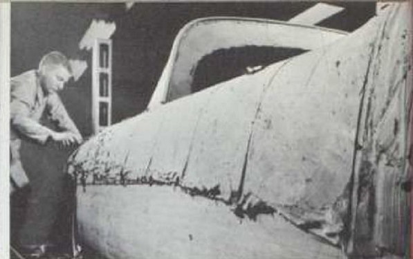
Series of contour lines at belt line just before excess clay is cut away.
