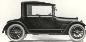
Convertible Victoria with windows lowered and pillars removed
